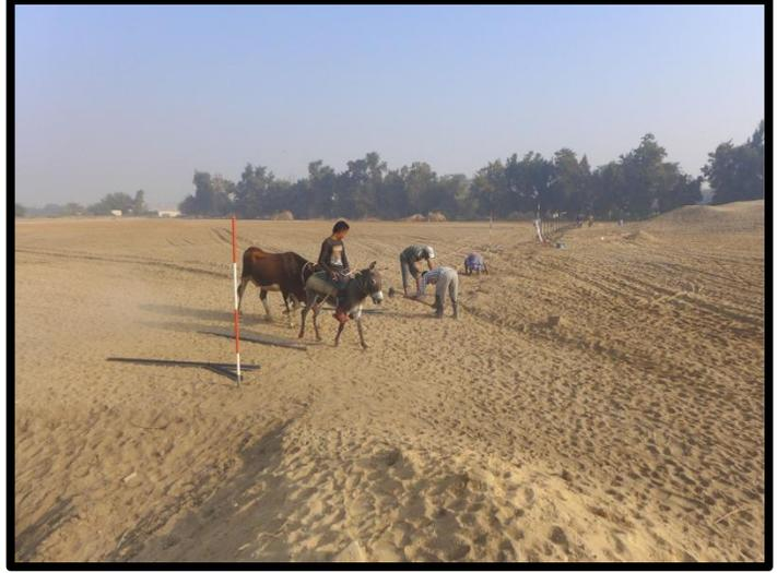
**Figure 3:** Survey line for the fence.
