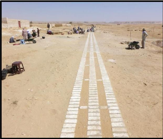
**Figure 19.** The foundations are made to be flush with the present surface of the desert. In the future they will be covered by a single course of blocks of fine Tura limestone cut to the ancient block size.
