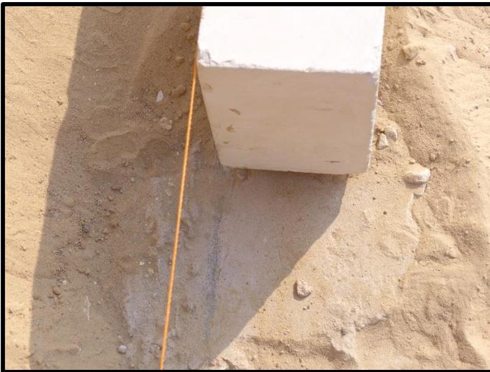
**Figure 17.** A patch of the gypsum-concrete foundations still preserving the original builder's ink guide line. A layer of sand is being used to cover it but, for the moment, the line is exposed to allow the modern builder's line exactly to follow it.
