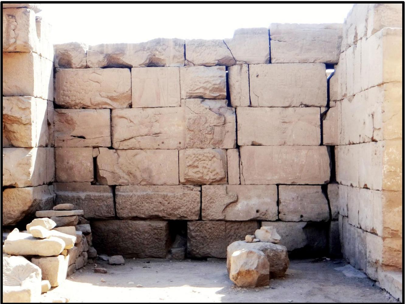
**Figure 8:** Luxor temple, the rear wall of Room XVI. The outline of the dividing wall, the raised floor and cavetto cornice are preserved from how the builders dressed the surface of the sandstone walls prior to carving the decoration. Photograph by Juan Friedrichs.
