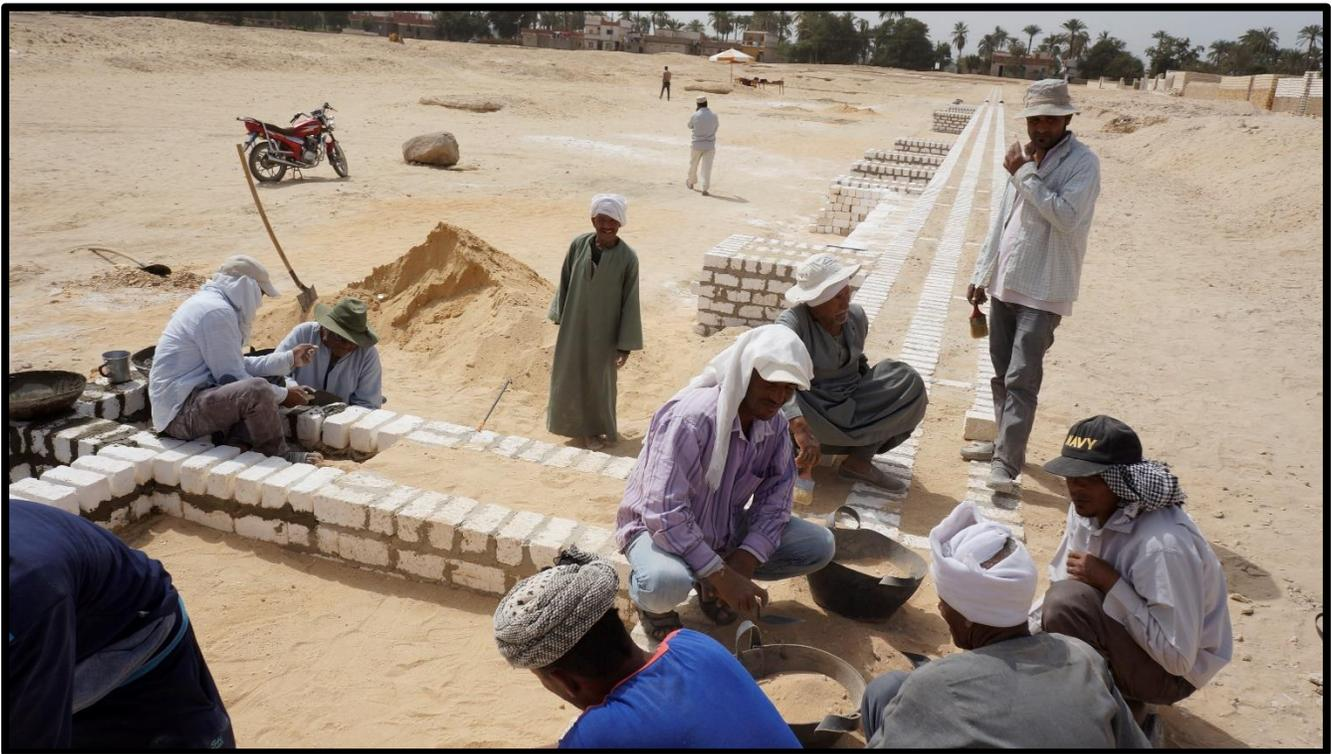
**Figure 5:** View to the west of the completed foundations for the final course of Tura limestone blocks along the line of the north wall of the Long Temple. The foundations run to the pylon at the front of the temple. The wall under construction in the foreground is the side of one of the small rooms, each of which contained a single offering-table, visible at a later stage in Figure 15. The large granite boulder discussed in the text stands in front of the motor-cycle.
