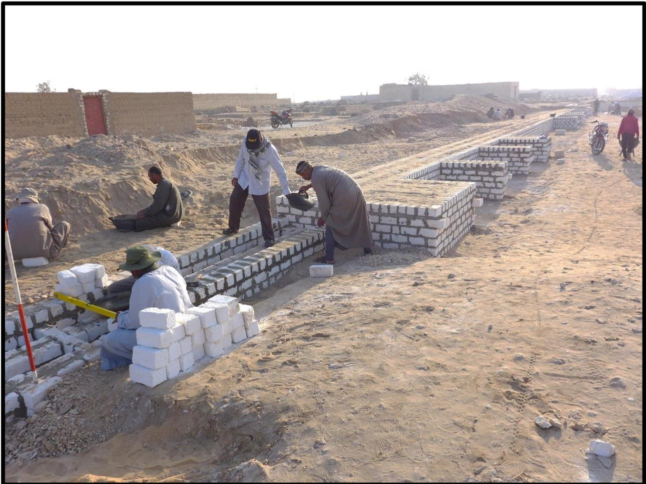
**Figure 3:** View of the same area as Figure 2 but viewed to the north-east and after the new stone foundations had been nearly finished. The thick projections added to the main wall represent the beginnings of walls which cross the temple from side to side. When the intended scheme is finished, none of the small blocks will be visible.
